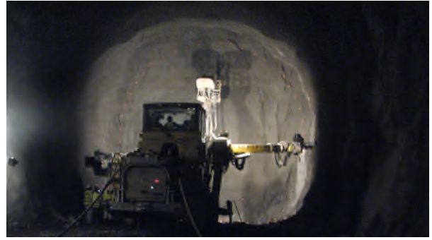
Drill and blast at the turbine tail race tunnel at Salomonde II site
